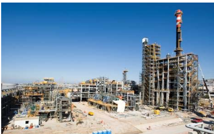
Thessaloniki refinery upgrade
